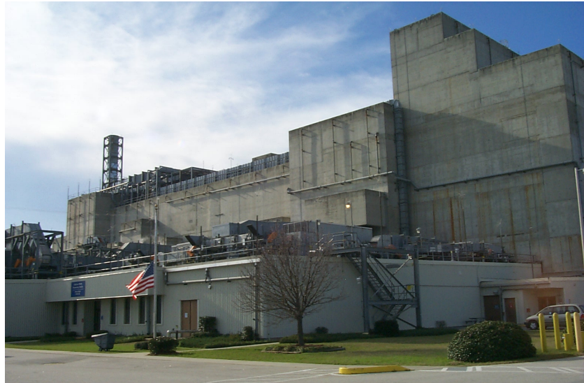
The Defense Waste Processing Facility safely immobilizes radioactive waste by mixing it with molten glass and then pouring the mixture into stainless steel canisters that are welded shut.
