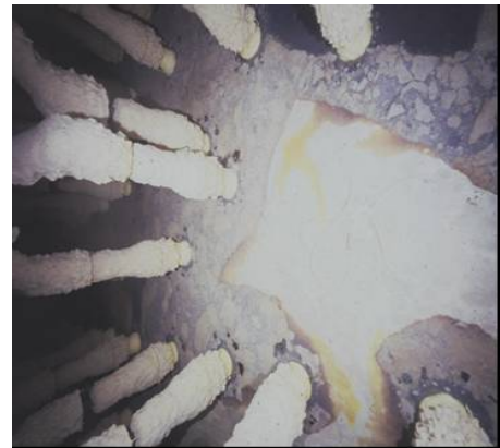
Salt cake forms in the waste tanks, taking up most of the room inside the tanks.
