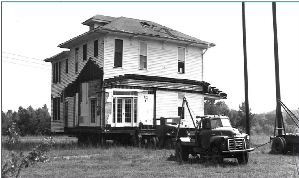
Figure 1 Relocation of House during SRS Construction
