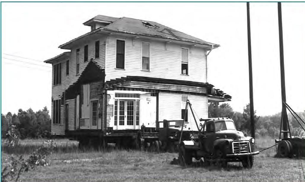
**Figure 1 Relocation of House during SRS Construction**
