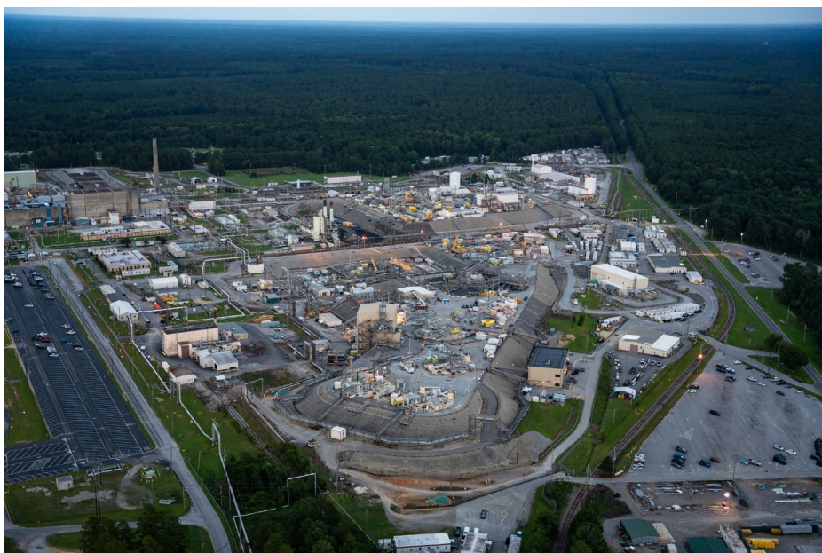
A record amount of radioactivity has been reduced over the last two years in waste tanks at the Savannah River Site.
