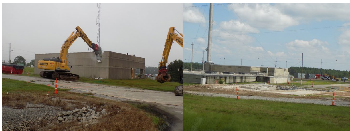
Before and after photos show the successful demolition of the 720-F Central Alarm Station down to a slab.
