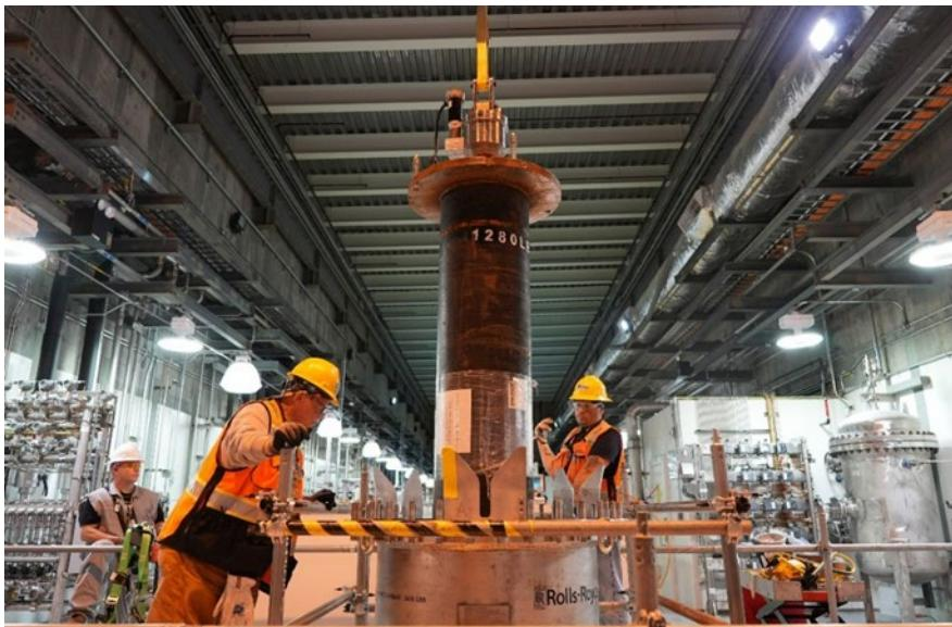
*Savannah River Mission Completion installed three larger, higher-capacity cross flow filters used in the decontamination process at the Salt Waste Processing Facility to achieve the facility's optimum production rates. Pictured are personnel conducting a mock-up trial of the filter changeout before executing the work in a highly radioactive area.*
