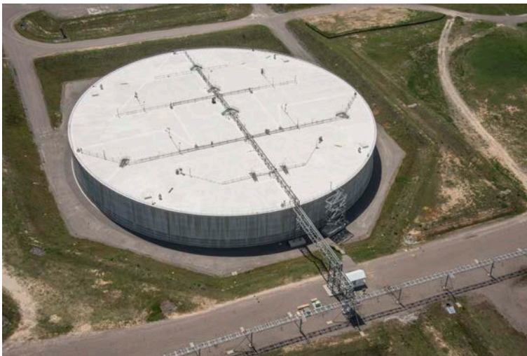
Savannah River Site's first mega-volume Saltstone Disposal Unit sits on 2-1/2 acres and will hold about 33 million gallons of saltstone.
