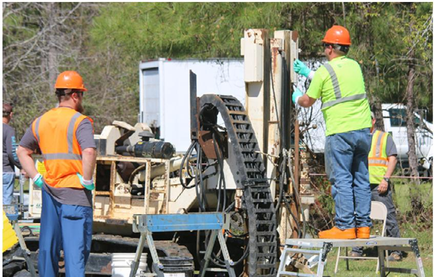
*Savannah River Nuclear Solutions (SRNS) radiation control inspector Ian Reed, left, observes Josh Justice, a driller for SRNS subcontractor Cascade Drilling, during the installation of an injection well for the silver chloride at SRS.*
