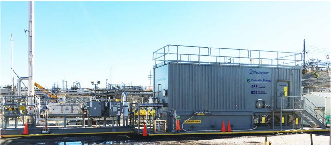
**Cutline 1:** The TCCR unit, stationed near Tanks 10 and 11 in the SRS H Tank Farm, consists of three modular skids: a main process enclosure housing all systems and components to treat the radioactive salt waste, a separate ventilation skid to provide environmental conditioning and contamination control for the main process enclosure, and a control skid to house the operating and video monitoring systems and provide for operator interface.
