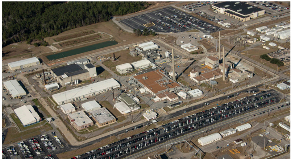
Aerial of the tritium facilities at SRS.
