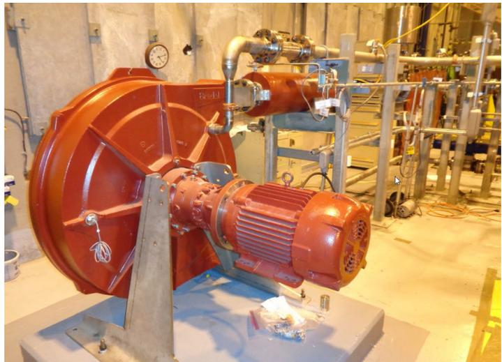
*Savannah River Remediation (SRR) made significant improvements to the Saltstone Hopper Overflow Container at the Savannah River Site's Saltstone Production Facility. Pictured is the container's recovery pump, foreground, with piping and additional new equipment as part of the facility improvements.*
