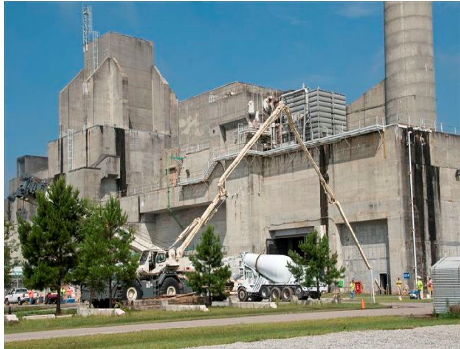
Grouting at P Reactor
