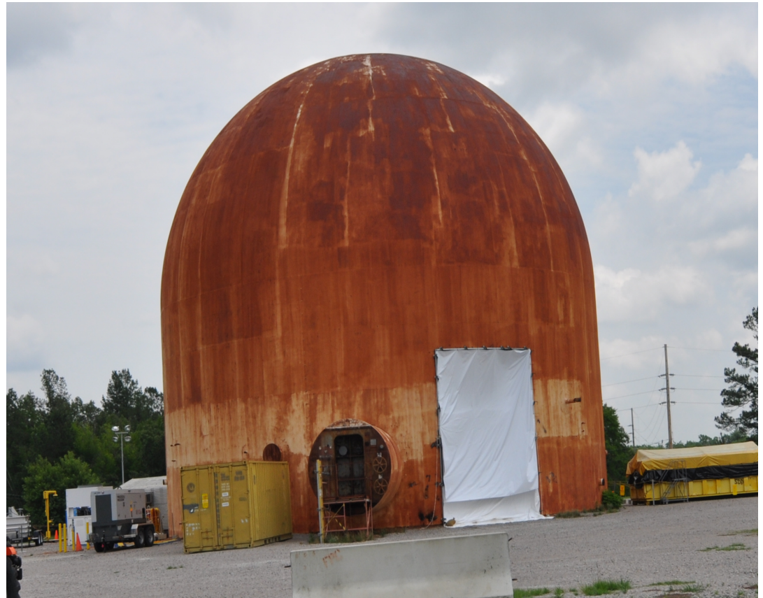
D&D Crews completed cutting a second access door
