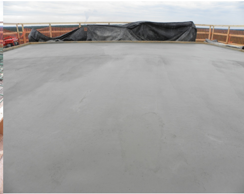
Final roof cap after curing at +149
