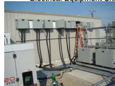
Connecting the tank pumps to Electrical Equipment Skid
