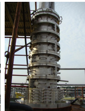
Installing the pump into the tank
