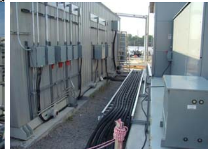
Installing the Electrical Equipment Skid on pad
