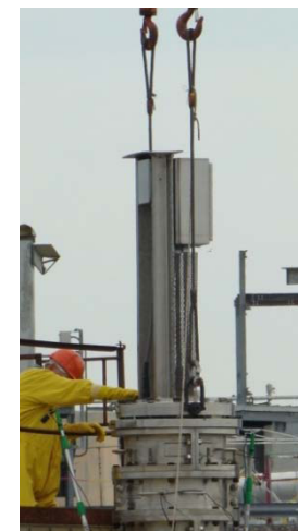
Installing the pump into the tank
