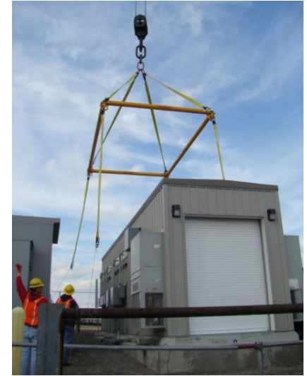
Installing the Electrical Equipment Skid on pad
