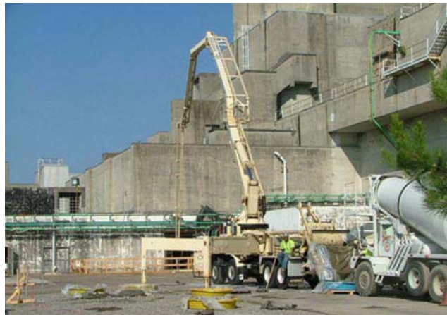
Specially engineered grout fill being pumped into a P Reactor building.
