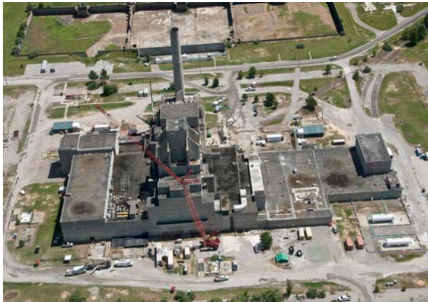
P Reactor at Savannah River Site Undergoing In-situ Decommissioning
