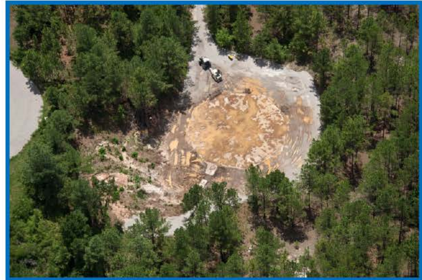
C Area Emergency Retention Basin (after)
