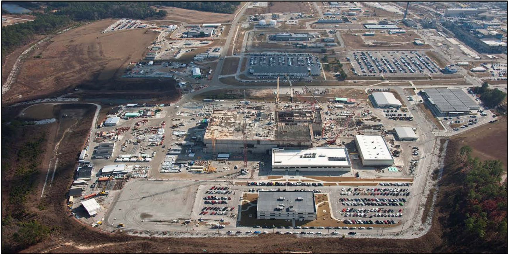
MOX Construction Site – December 2012
