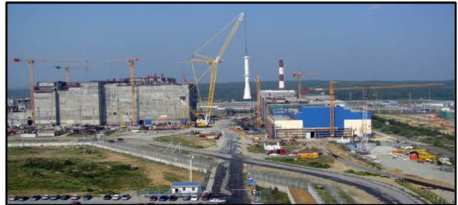
Construction of the BN-800 Fast Reactor, Beloyarsk, Russia
