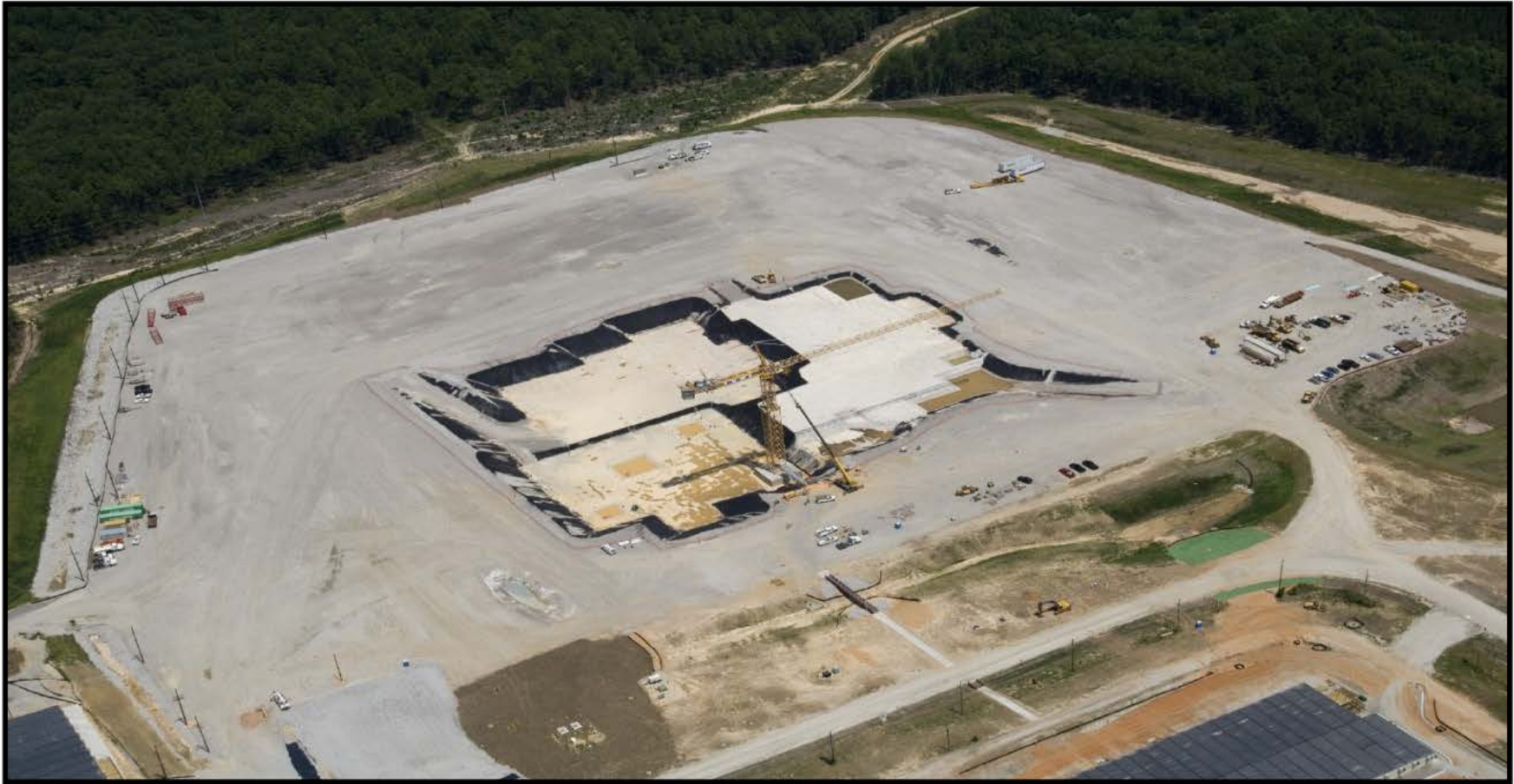
MOX Construction Site – July 2007
