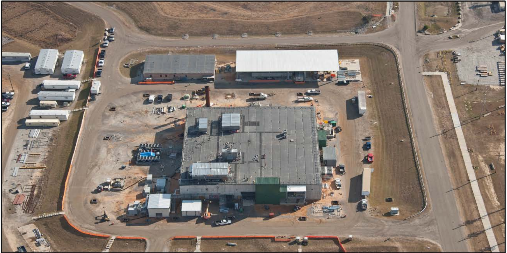
Waste Solidification Building – December 2012
