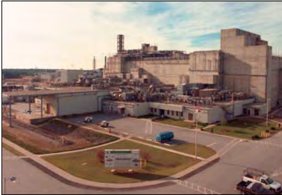
Defense Waste Processing Facility
