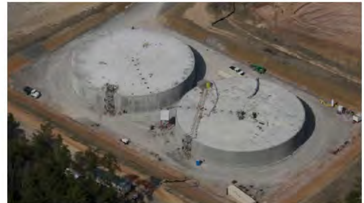
Salt Disposal Units
