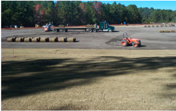
R Area Ash Basin
