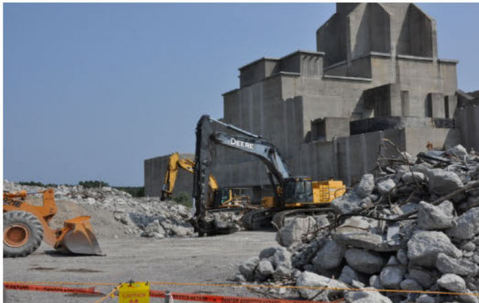
P Area Disassembly Basin
