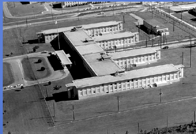
Administration Building after Completion
