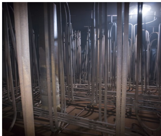
Tank 5 Cooling coils before sampling/grouting
