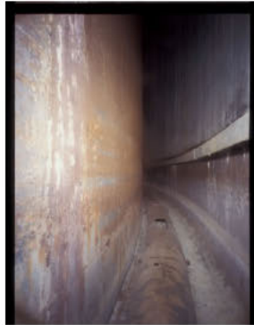
IP-35 View of SE
