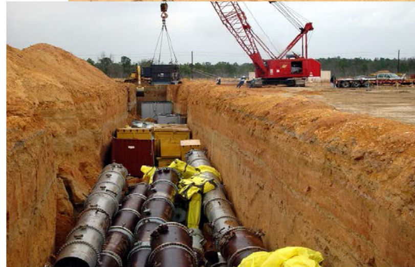
Two pictures of trench disposal
