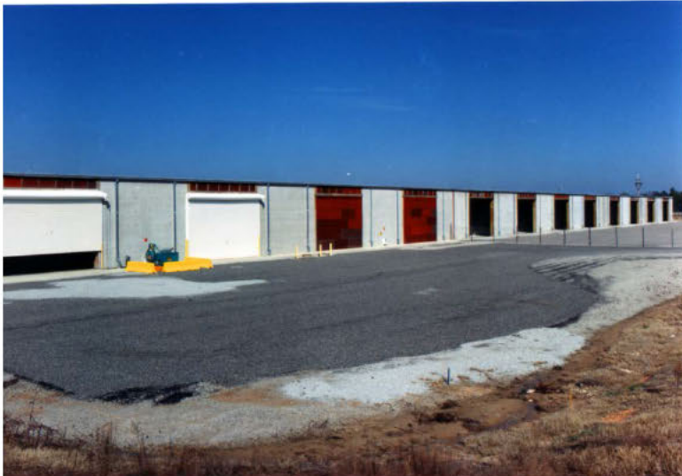
Low Activity Waste Vaults
