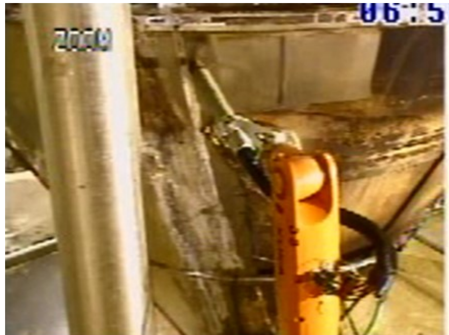
Picture taken during removal of the stainless steel-wrapped insulation on the cone of the evaporator pot
