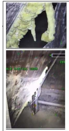
South Leak-site (the salt streak)
