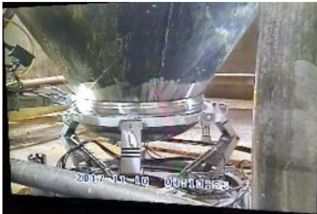
Robotic welding of cap to evaporator vessel
