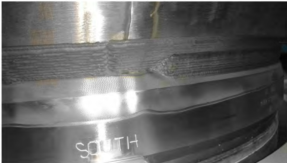
Figure 4 Several weld passes are needed to complete the installation (the remote welder removed to show the weld passes in progress)
