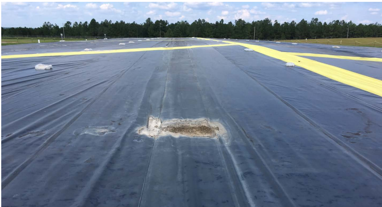
Figure F-8. Subsidence of Intact Covers (~1.5 m [5 ft] diameter) at Slit Trench Disposal Unit 5 (2016)
