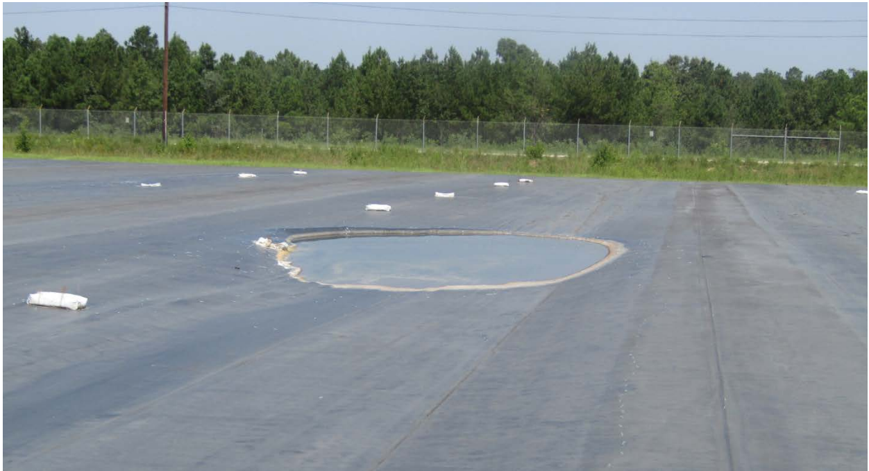
Figure F-7. Subsidence of Intact Covers (~3 m [10 ft] diameter) at Slit Trench Disposal Unit 4 (2016)
