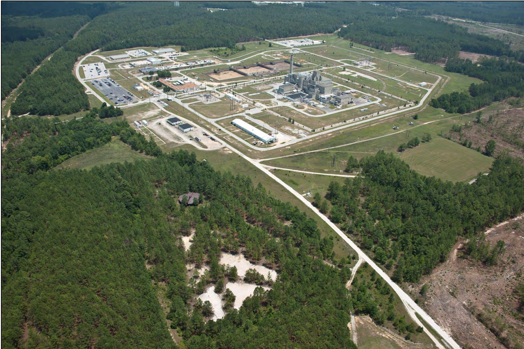
Figure C-2. Aerial Photograph of CAOU (2011)
