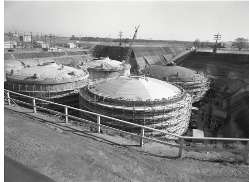
Many of the waste tanks at SRS were built in the 1950s.
