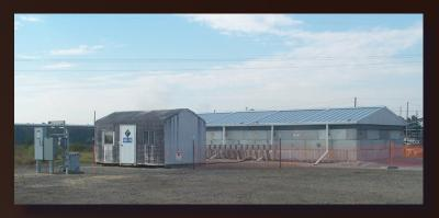
Above: A thermal detribution unit is seen in the background, with the switchgear and control room seen in the foreground.
