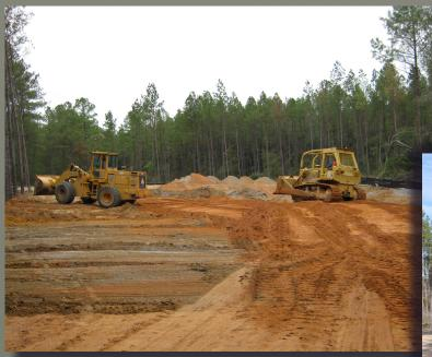
Above: The ECODS B-3 & B-5 were backfilled and graded for mechanical completion.
