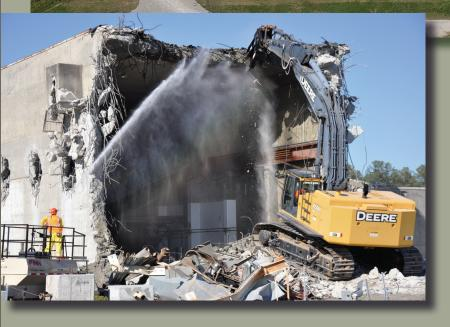
The stack removal (above, right) and disassembly basin demolition (left) in R Reactor (above left) were two activities that have brought the building closer to final closure.
