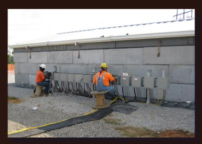
Above: SRS workers complete the electrical connections to the thermal detritiation unit heating elements.
