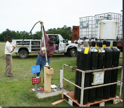
The edible oil is deployed in a well in SRS's T Area by ACP employees, which has been shown to reduce the amount of cVOCs in groundwater plumes.
