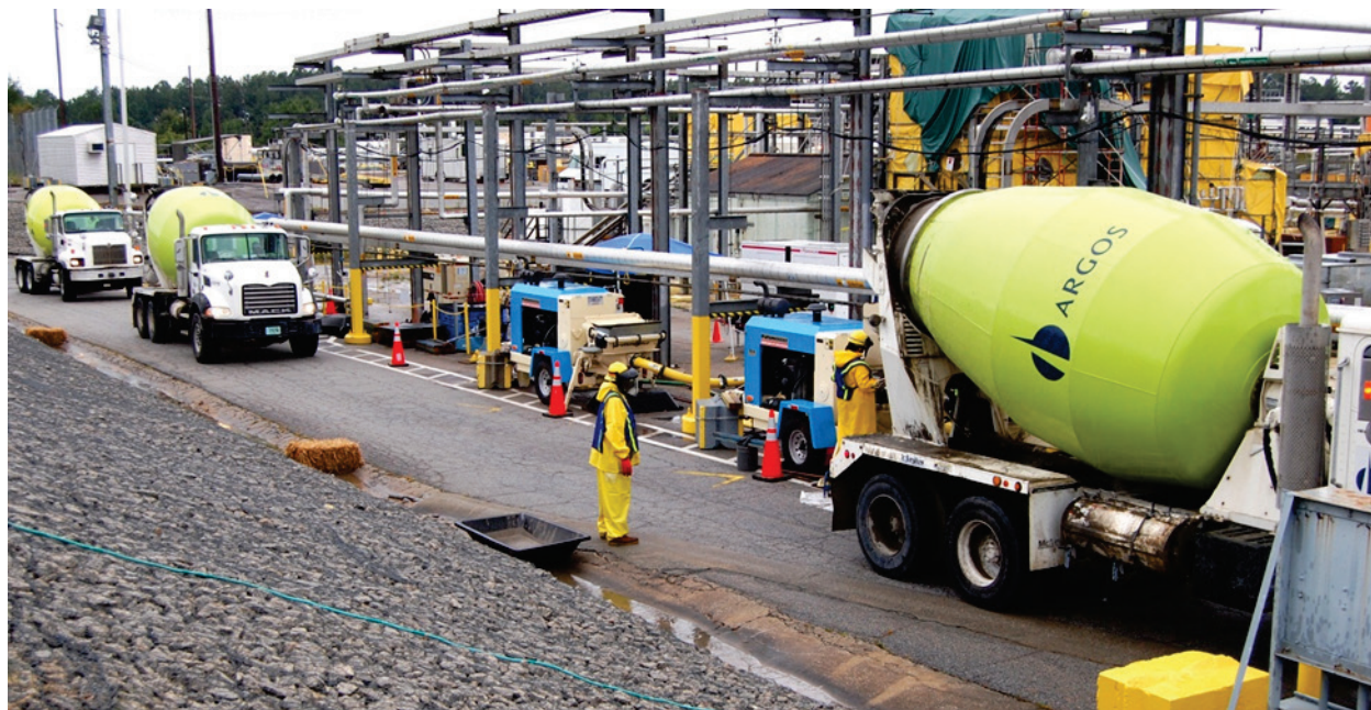
Figure 3-1 SRS Employees Grouting Tanks 5F and 6F
