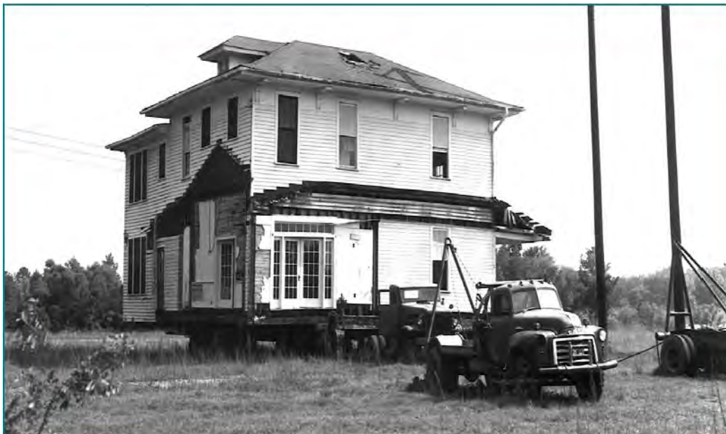
Figure 1 Relocation of House during SRS Construction
