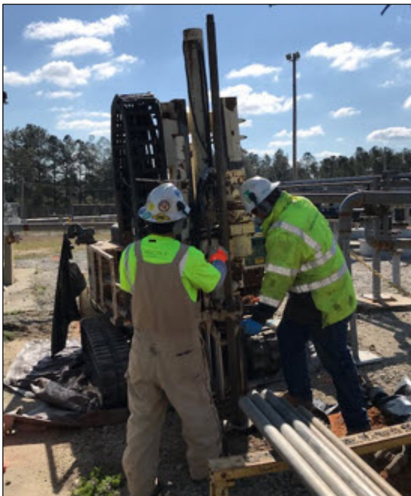
Soil Sampling at the Solvent Storage Tanks
