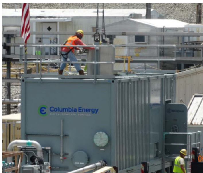
Ion Exchange Column Installed at TCCR
