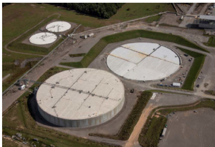
Saltstone Disposal Unit (SDU) 7 Being Constructed Next to SDU 6
