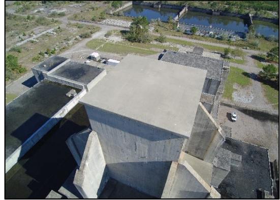
Drone's View of P Reactor
