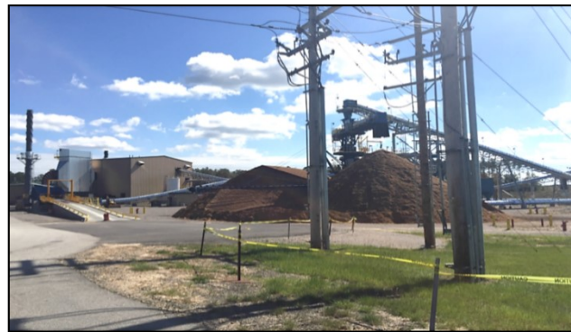
Biomass Cogeneration Facility
