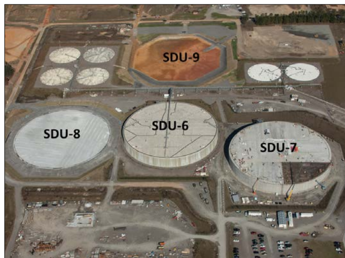
Saltstone Disposal Units Being Constructed Next to SDU-6
