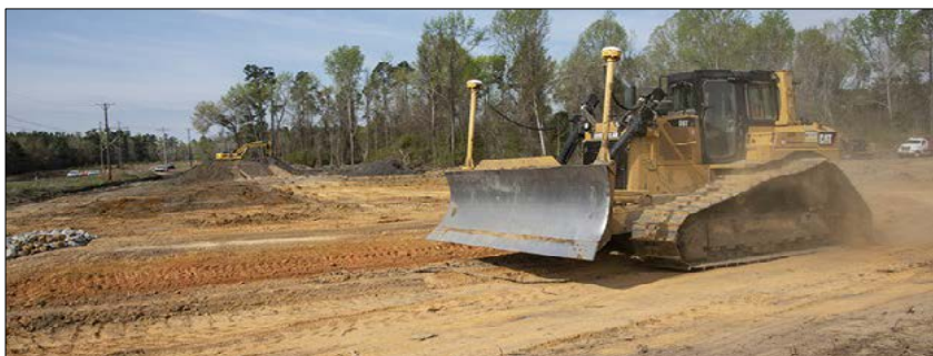
Work in Progress at Wetland Area at Dunbarton Bay
