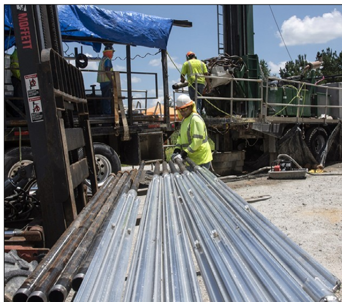
Installing P-Area Groundwater Remediation Technology
