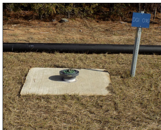
Flange on Injection Well Head
