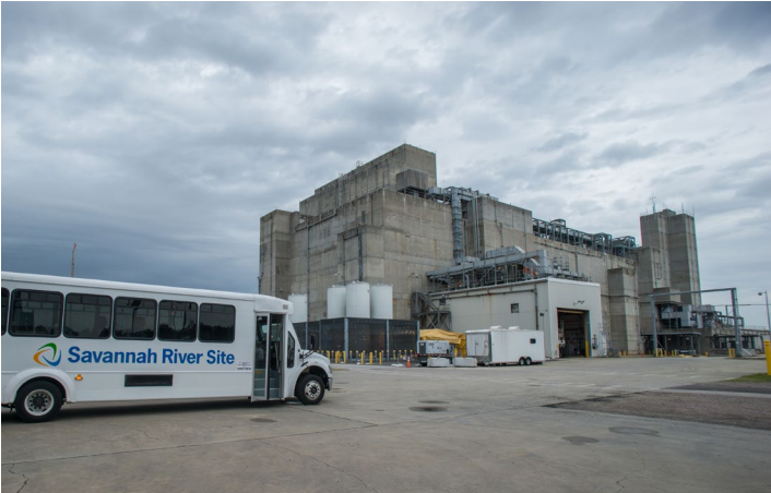
The Defense Waste Processing Facility processes the sludge, mixing it with borosilicate glass at 2,100 degrees Fahrenheit.
