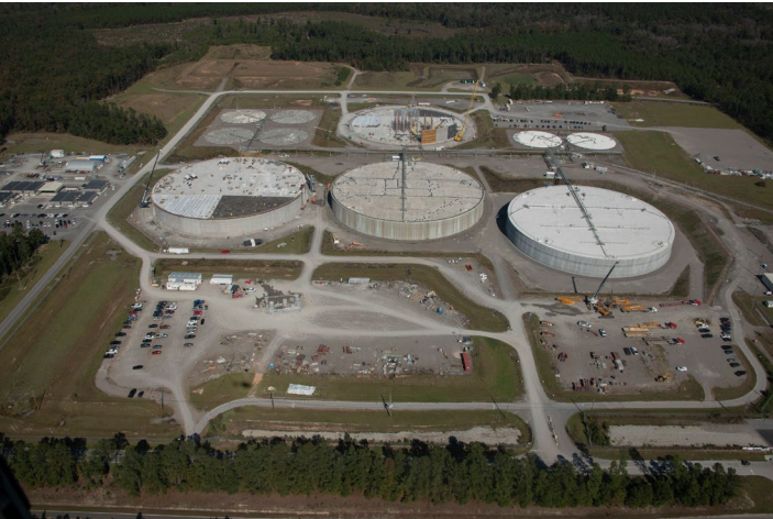
By the end of 2021, two of the 32-million-gallon mega-vaults were completed, and another two were in progress.
