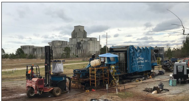
A Subcontractor Loads Zero-Valent Iron Filings during Injections to Support Installation of the P-Area Reactive Barrier
