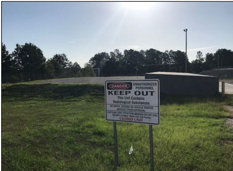
Final View of the SSTs
