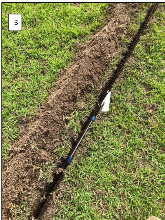
Figure 3-4 Installation of ERT Electrode Cables
