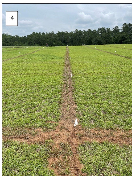
Figure 3-4 Installation of ERT Electrode Cables
