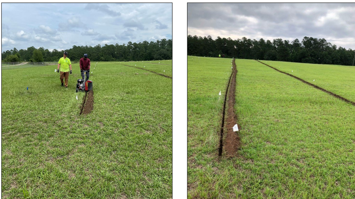
Figure 3-3 Trench Installation to Bury Electrode Cables
