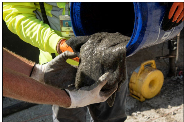
Zero-Valent Iron Filings Undergo Preparation Before Being Injected into Wells during the P-Area Reactive Barrier Installation.
