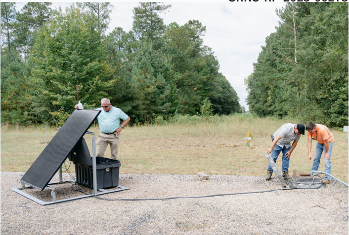
Savannah River Nuclear Solutions’ Site Services employees inspect the D Area solar-powered pump system that manages water infiltration in underground valve pits at the Savannah River Site.
