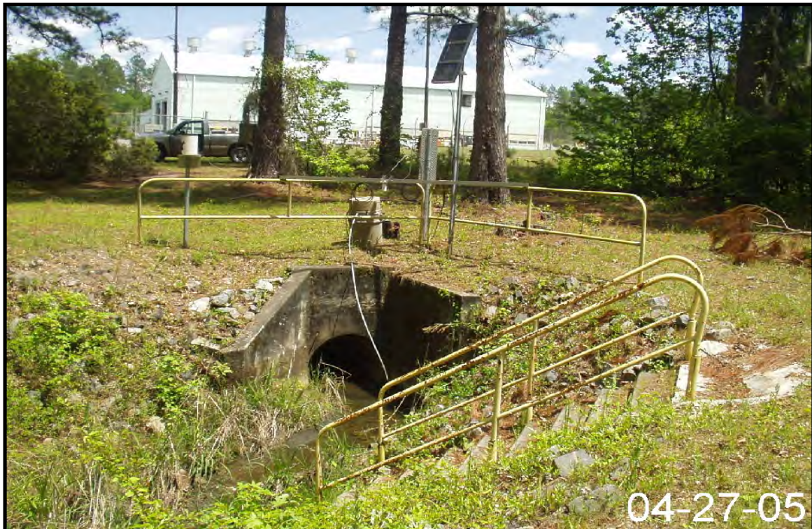
Figure 2-120. View of Stormwater Outfall Y-01.
