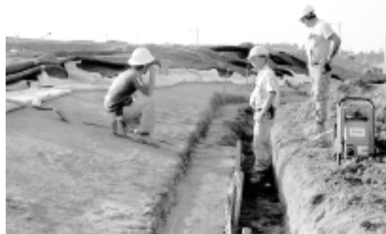
Workers survey anchor trench at engineered low-level trench #4.
