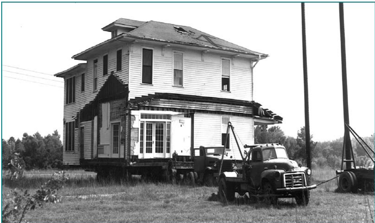
Figure 1 – Relocation of House During SRS Construction
