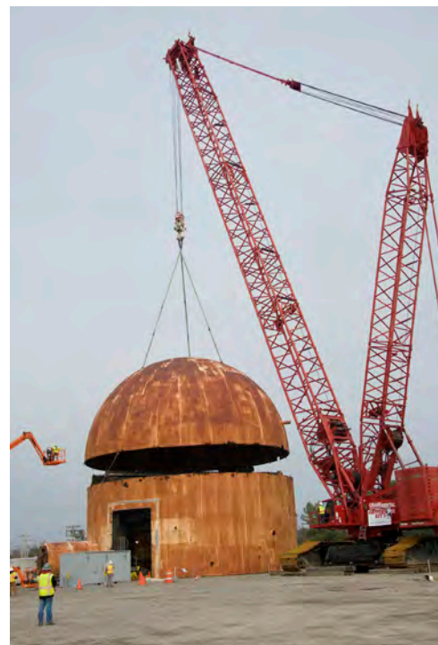
A giant crane slowly lifts the dome from the Heavy Water Components Test Reactor, an SRS landmark since 1959.
