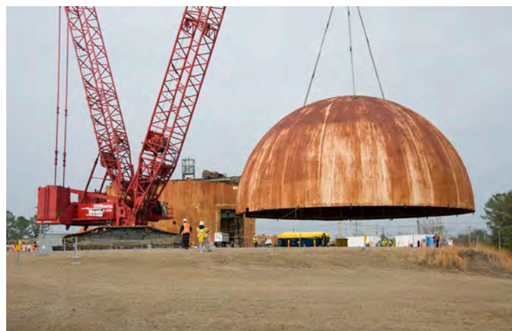
The dome of HWCTR is slowly and safely lifted and lowered to the ground.
