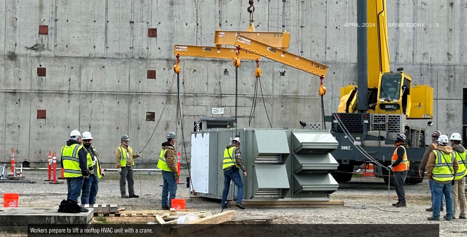
Workers prepare to lift a rooftop HVAC unit with a crane.
