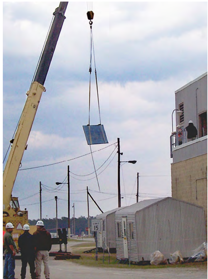
A crane performs a critical lift to replace a heavy heating and cooling coil that was damaged in the January 2014 sub-freezing temperatures.
